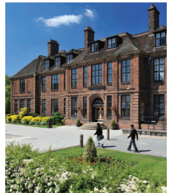
The Venn Building, Hull Campus
